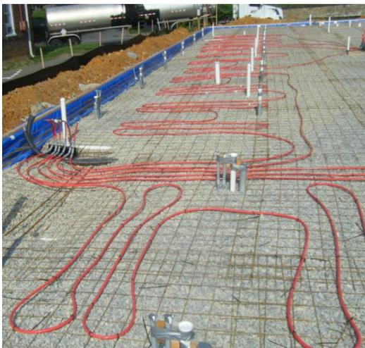
Figure 2 - Passive Radiant Cooling Rough-in
